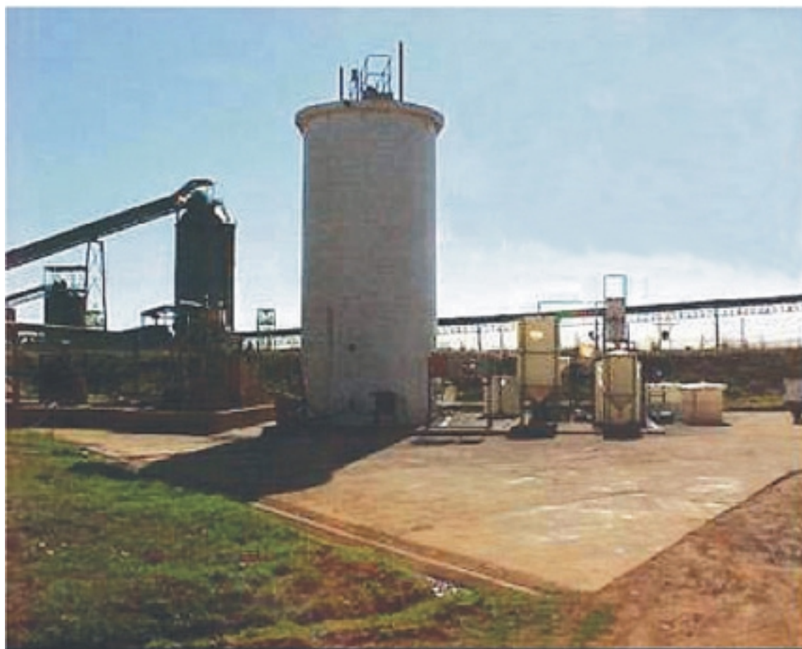
Figure 4-7: Anaerobic Bioreactor Employed for Sulphate Removal
